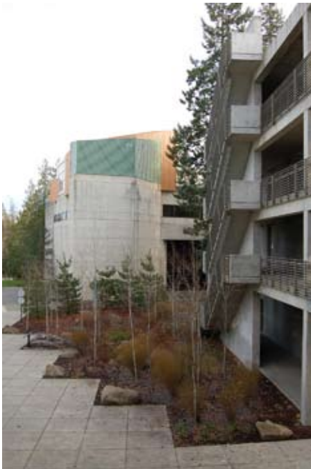
Seminar II building uses bioswale technology for storm water management.
